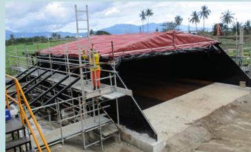
**IMAGE 2:** Full-scale Hottpad system. Processing rate is a function of the base size which can be increased by adding Hottpad modules.
