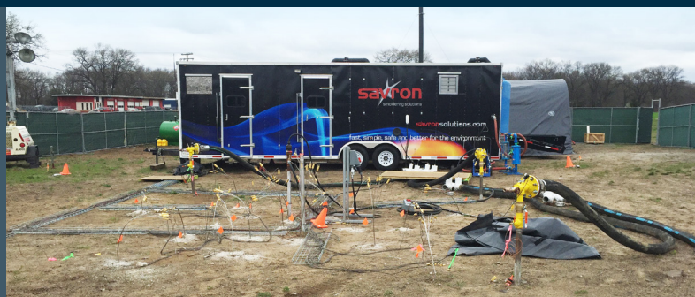
Figure 1: PDE test area showing the ignition/air injection well, associated thermocouple network, and the STAR control trailer.
