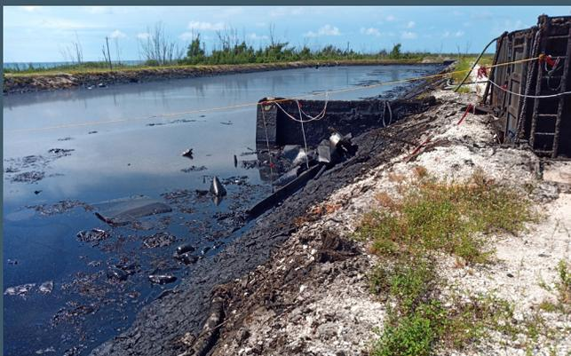
**IMAGE 2:** Oily sludge holding pond scheduled for closure. Sludge will be excavated and mixed with a porous matrix prior to smoldering in a STARx Hottpad™ system.
