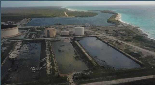
**IMAGE 1:** Oil and gas terminal in the Bahamas, showing the condition of the oily sludge holding ponds following hurricane Dorian.
