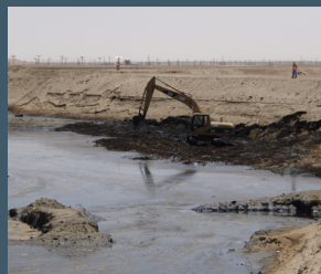
IMAGE 2: Excavation and consolidation of crude oil sludge
