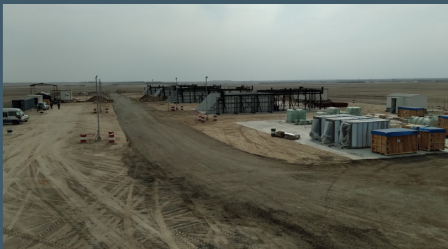
IMAGE 1: STARx Hottpad system under construction
