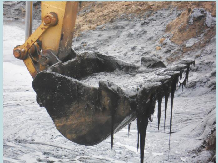
**IMAGE 3:** Oily sludge designated for treatment via STARx Hottpad™
