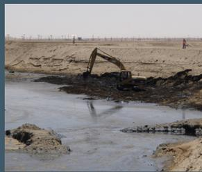
**IMAGE 2:** Excavation and consolidation of crude oil sludge
