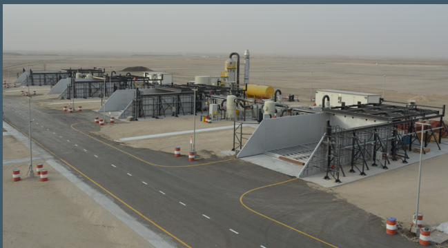
IMAGE 1: STARx Hottpad system under construction
