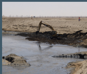
IMAGE 2: Excavation and consolidation of crude oil sludge
