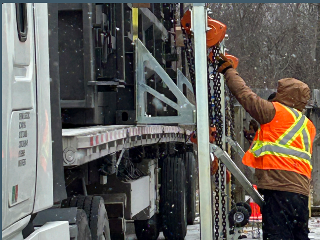
IMAGE 2: F35 vessel being offloaded from a truck
